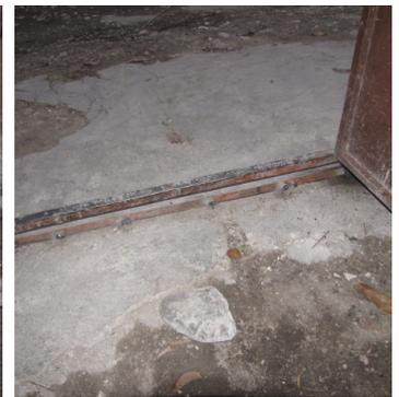
**Compound Front Gate:** The rollers were repaired/replaced and the bent rail track was straightened and secured
