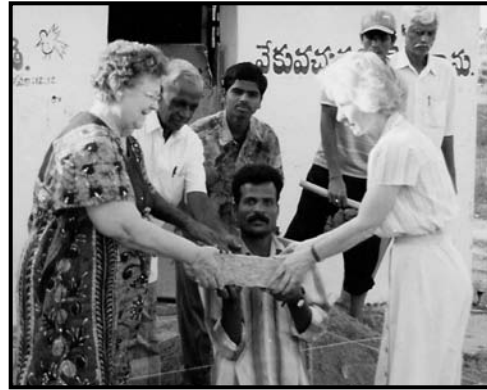
Geraldine (left) and Jan laying the first stone of the foundation for the new widow home.
